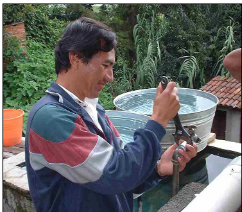
A community outreach worker in Mexico installs a UV tube developed by University of California, Berkeley researchers to purify water for individual households.
